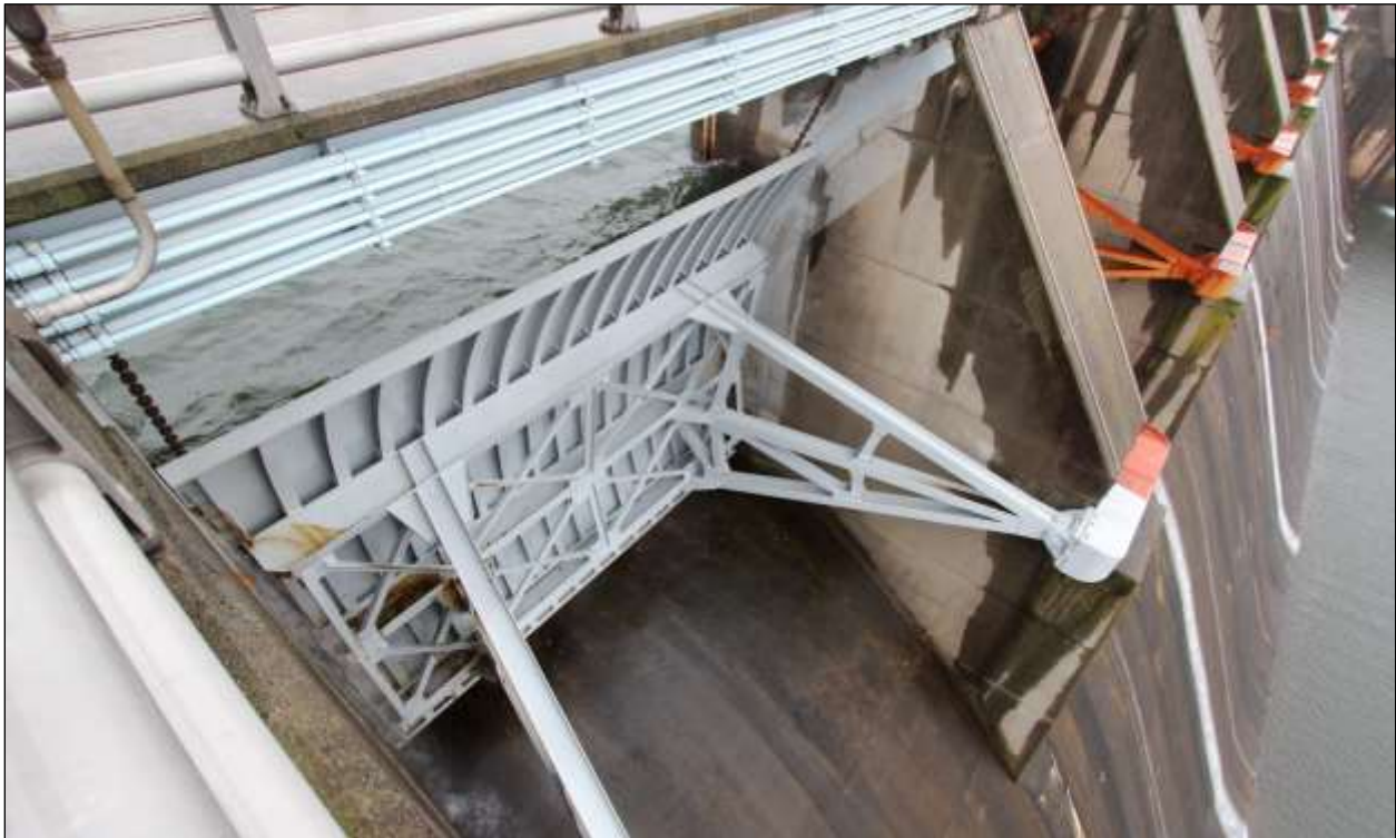
Figure 3.17. Cowans Ford Spillway, taintor gate.
