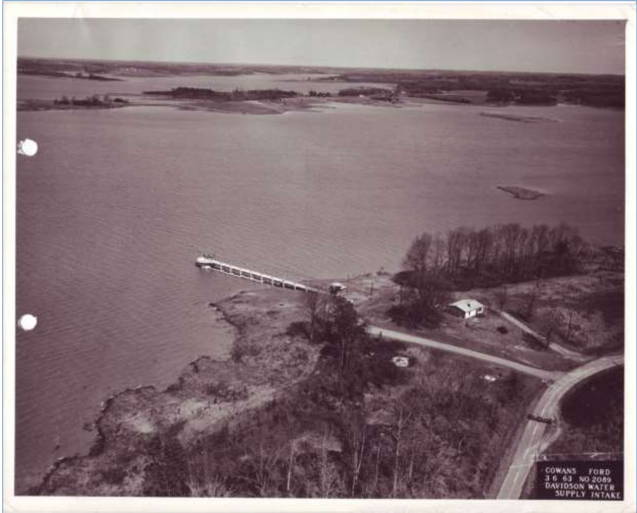
Figure 2.31. Some of the more necessary logistics for impounding Lake Norman included rebuilding intake systems for local municipal water supply. The one shown here is for the City of Davidson. Photo dated March 1963.
