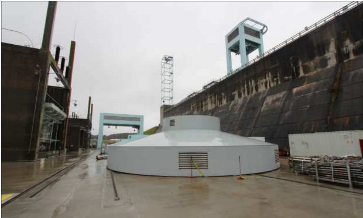
Figure 3.9. "Roof" of Cowans Ford Powerhouse, showing top casing of generating units. Transformers are in concrete casings at left.
