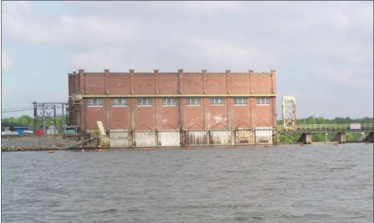
Figure 2.5. Lake Blackshear (Warwick) Powerhouse (constructed 1930), Crisp County, Georgia.
