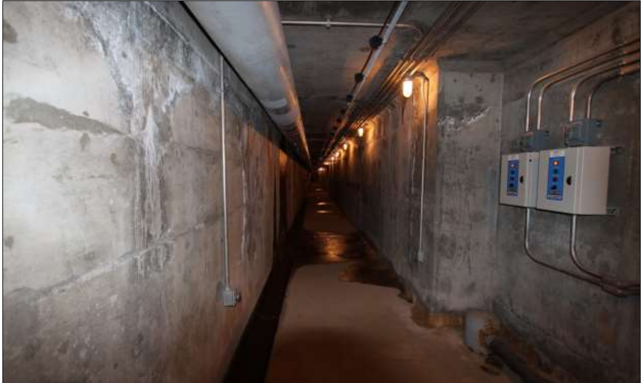
Figure 3.12. Inspection gallery in lowest level of powerhouse, facing east.
