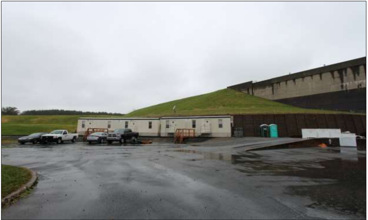
Figure 3.15. Cowans Ford Dam, east abutment.
