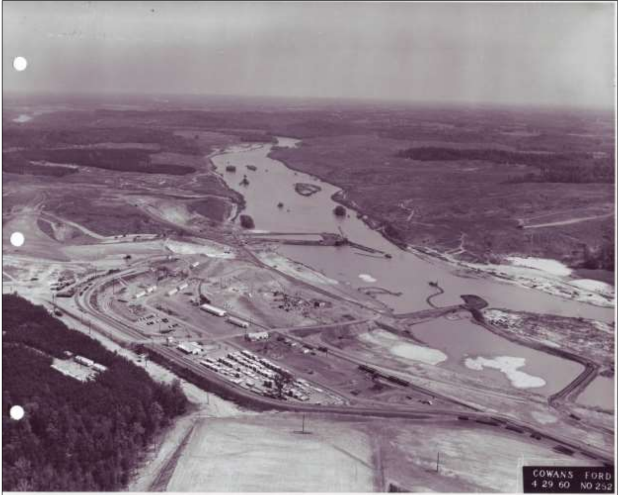
Figure 2.16. Cowans Ford, April 1960, showing early construction of coffer dam.
