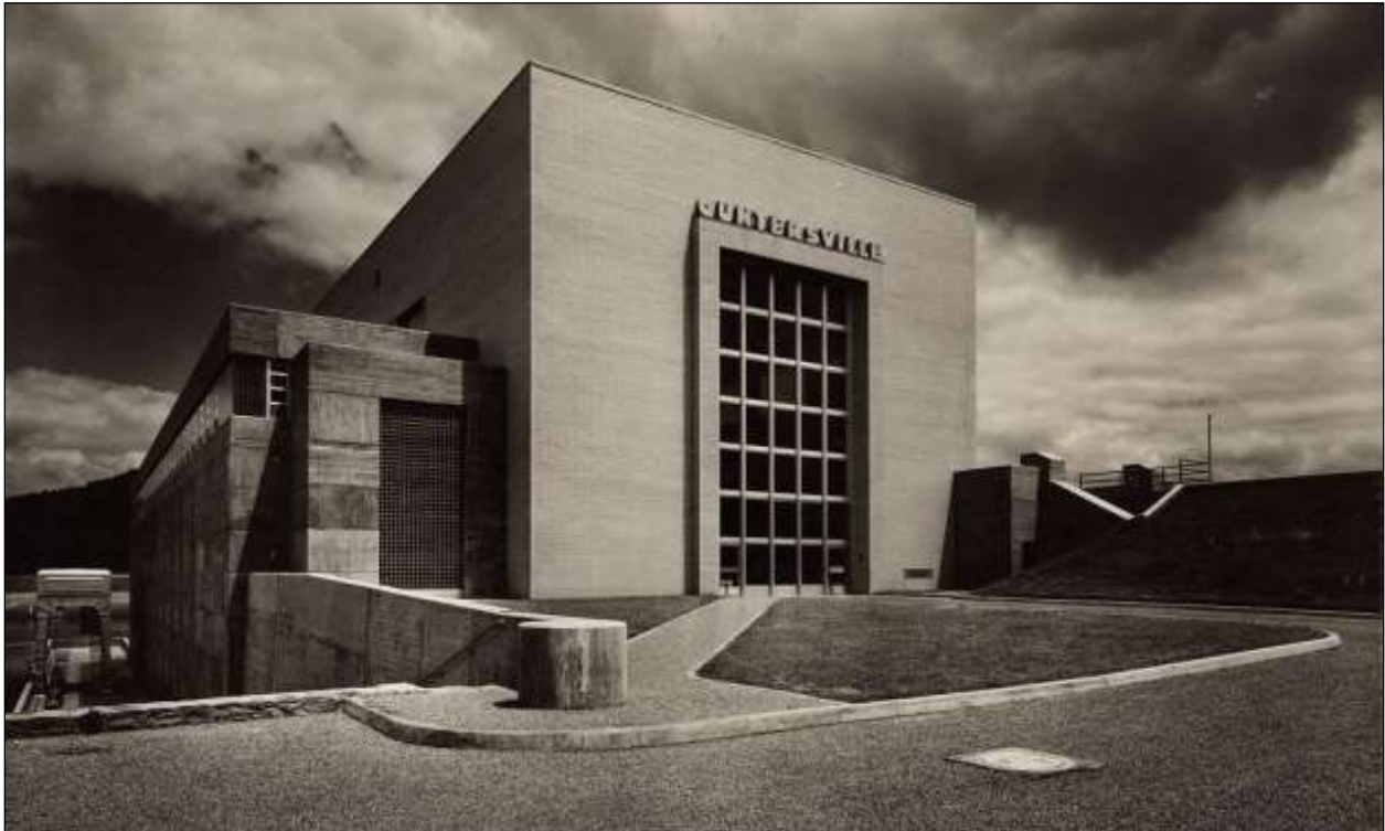
Figure 2.6. TVA's Guntersville Powerhouse (completed 1939), Marshall County, Alabama.
