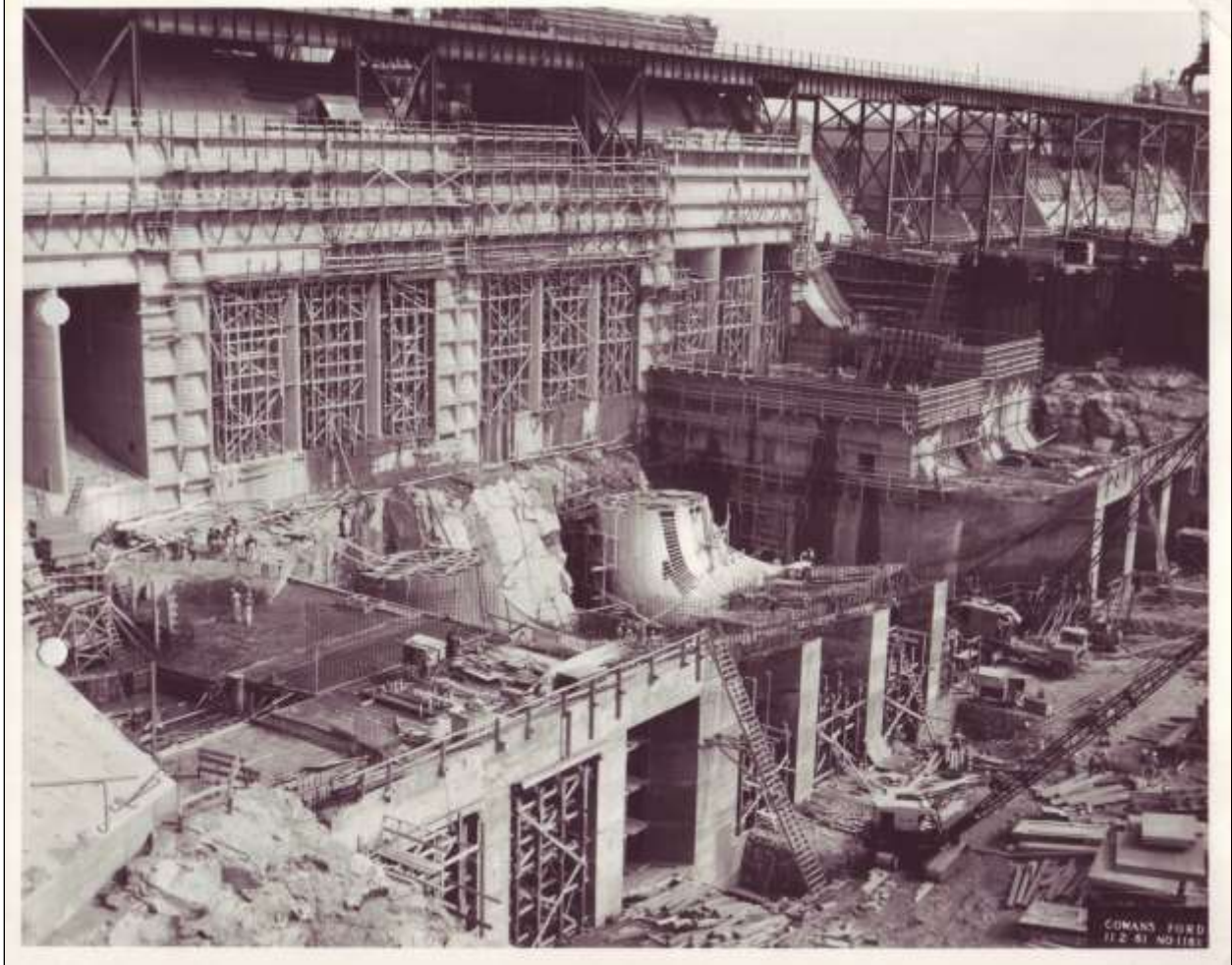
Figure 2.19. Cowans Ford Powerhouse, November 1961, showing construction.
