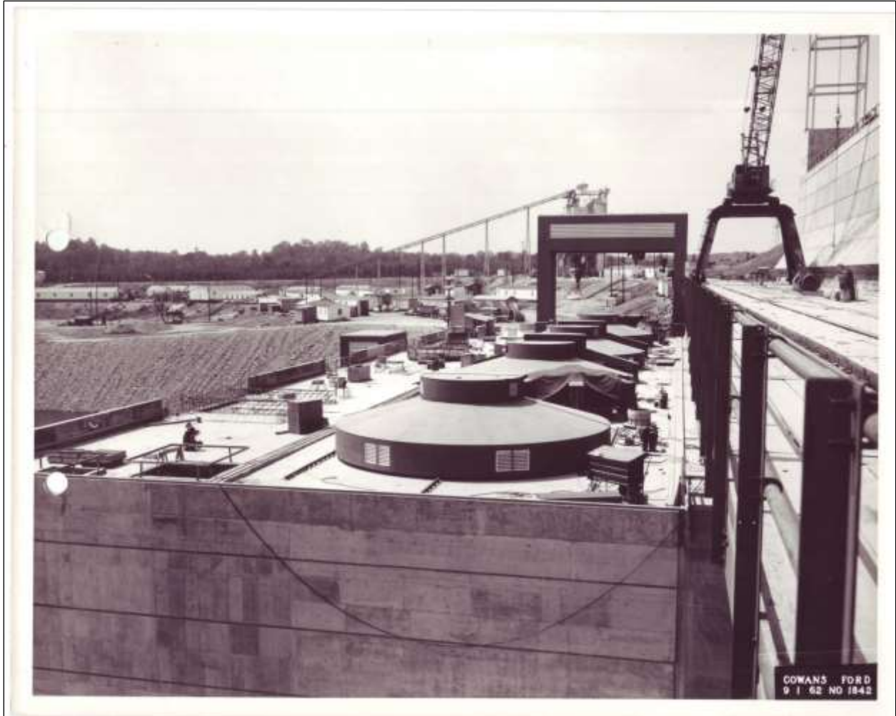
Figure 2.22. Cowans Ford Powerhouse, September 1962.
