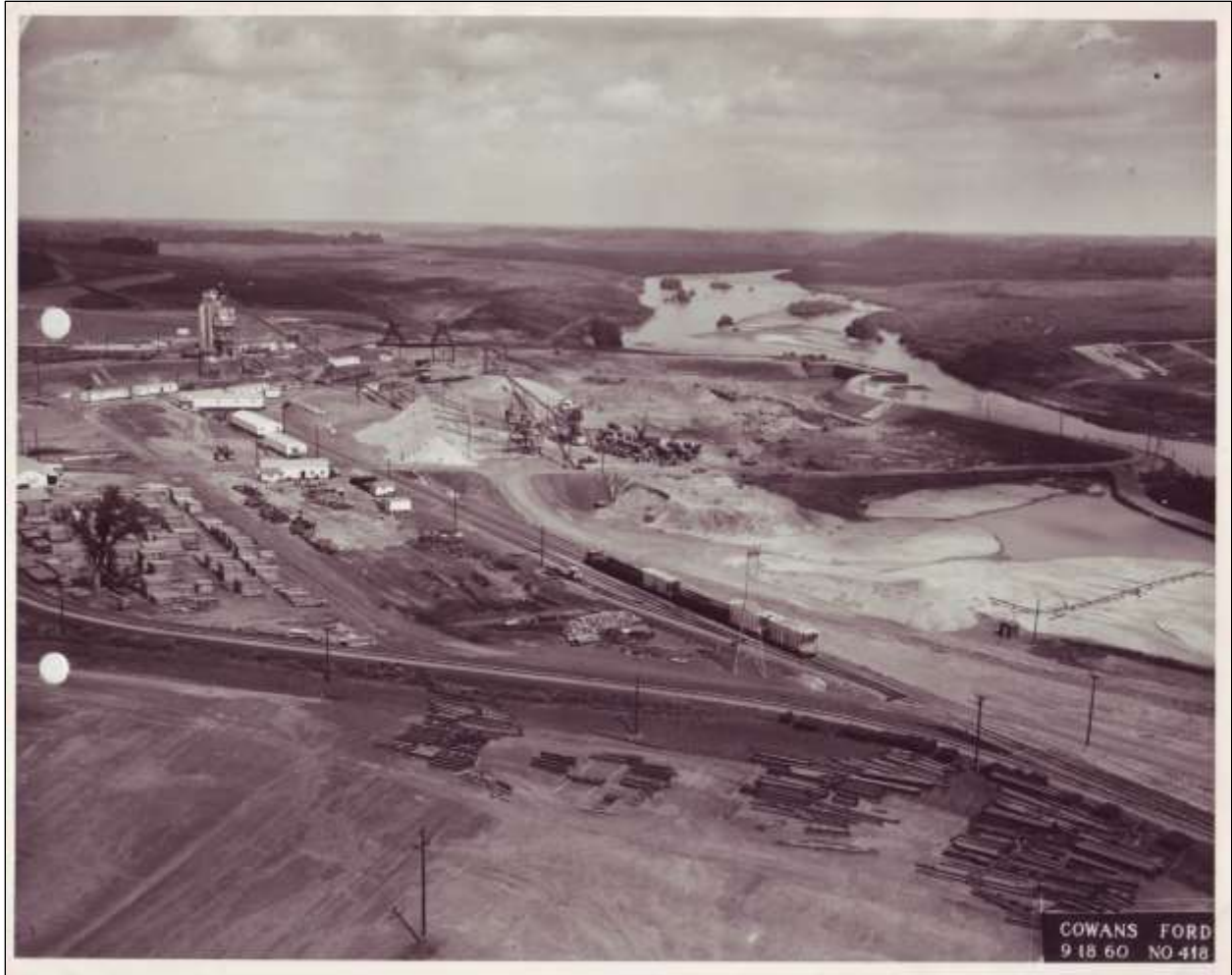
Figure 2.17. Cowans Ford, September 1960, showing manipulated river bed for construction.
