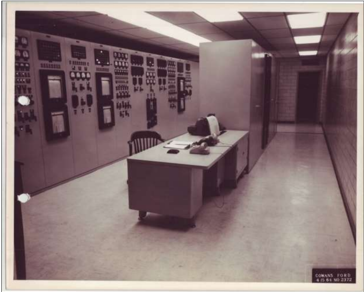
Figure 2.26. Cowans Ford control room ready for operations, April 1964.
