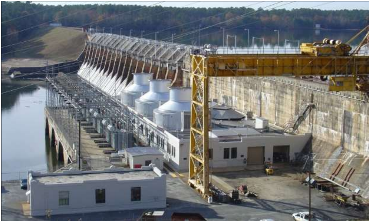
Figure 2.3. Semi-outdoor powerhouse design at the Tillery Development (completed 1928), Yadkin River, North Carolina.
