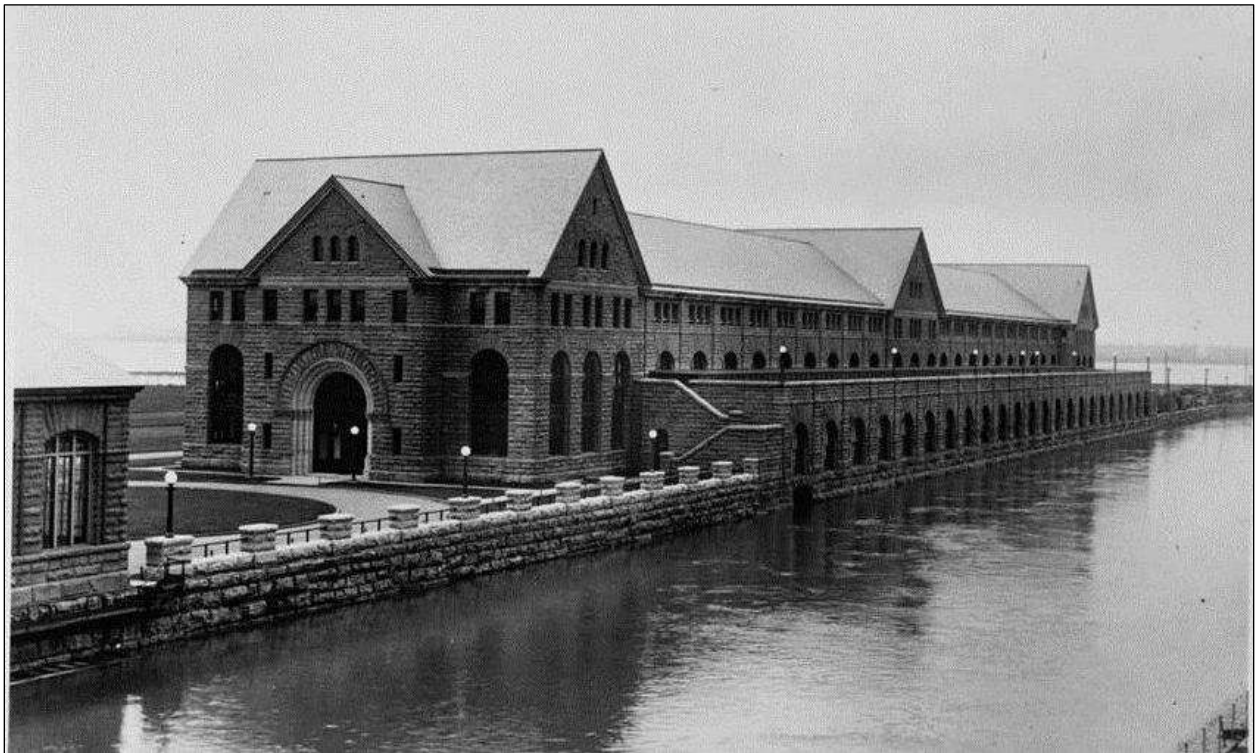
Figure 2.1. Adams Powerhouse (completed 1905), Niagara Falls, New York.
