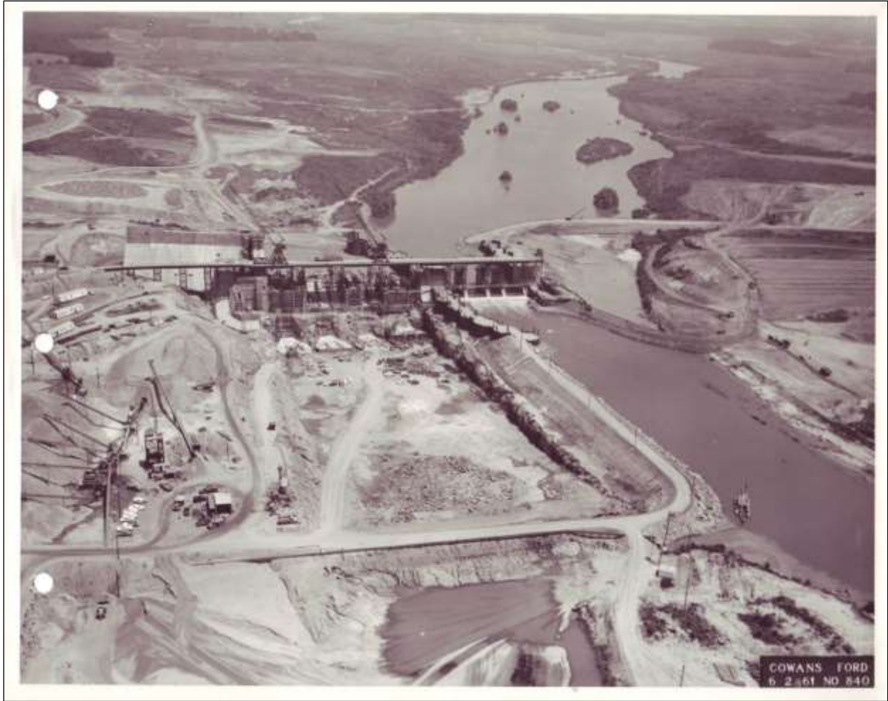
Figure 2.18. Cowans Ford, June 1961, showing water re-diverted back through gates.
