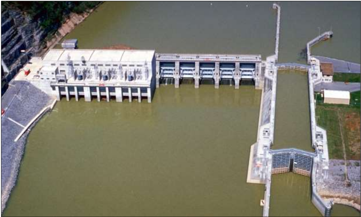
Figure 2.8. USACE Cordell Hull Powerhouse, Lock, and Spillway (completed 1973), Smith County, Tennessee.
