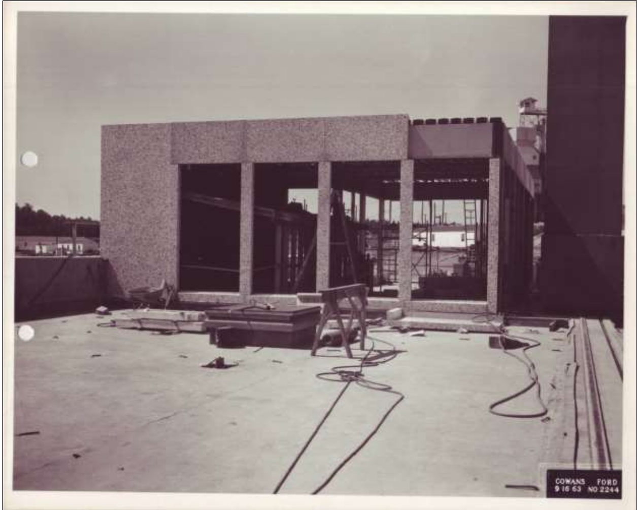
Figure 2.24. Cowans Ford Powerhouse entry, September 1963.
