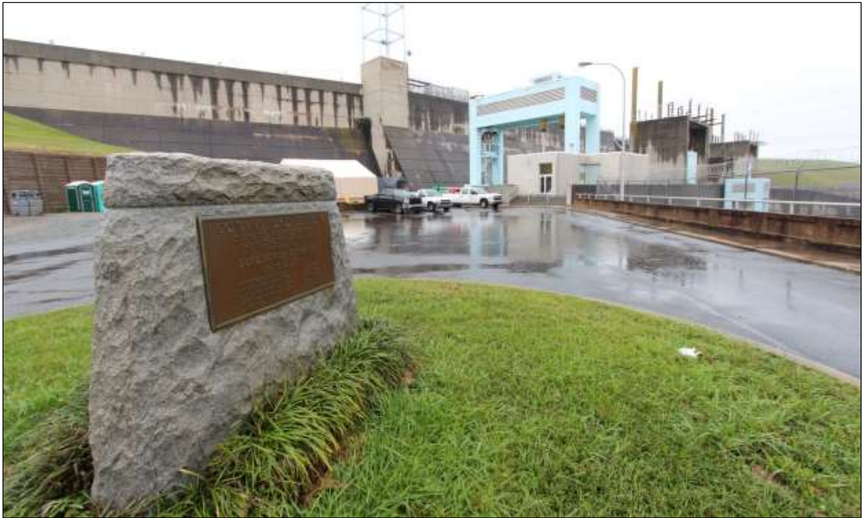
Figure 3.3. Cowans Ford Powerhouse and commemorative monument, facing northeast.
