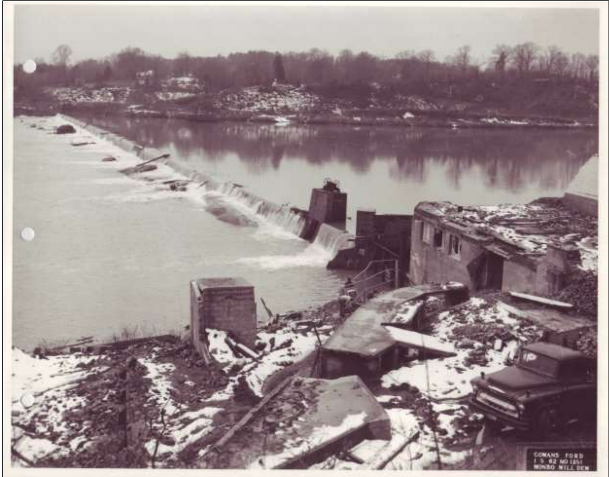
Figure 2.30. Impoundment of the lake required demolition and removal of several existing textile mill dams, including Monbo Mill. Photo dated January 1962.
