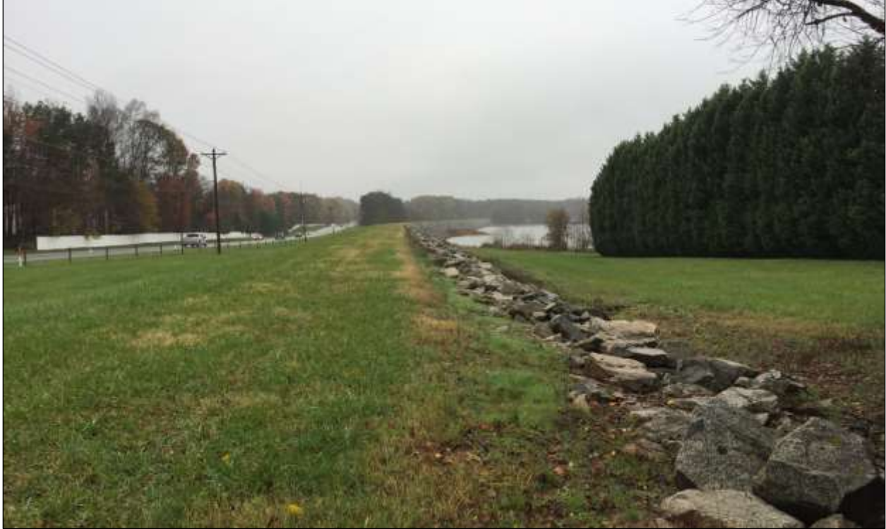
Figure 3.18. Hicks Crossroads Saddle Dike, facing northwest.
