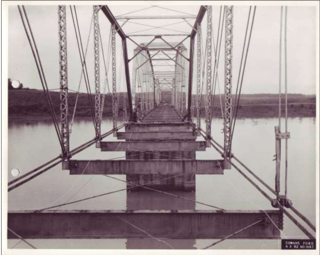
Figure 2.32. In this photo, dated June 3, 1962, Lake Norman is creeping up to the girders of the 1916 Beattie's Ford steel truss bridge, which carried North Carolina Highway 73 over the Catawba River. It was one of the last remaining obstacles in the Lake Norman impoundment.
