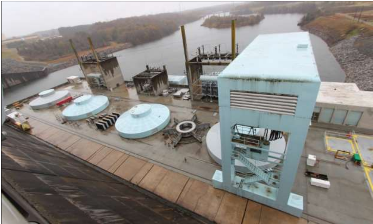
Figure 3.7. Cowans Ford Powerhouse, illustrating “semi-outdoor” design.
