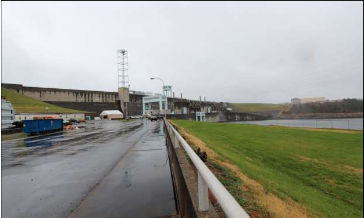
Figure 3.2. Cowans Ford Development, facing northeast.
