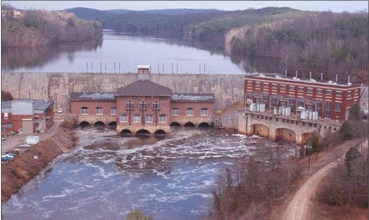
Figure 2.4. Duke Energy’s Great Falls-Dearborn Development, showing two phases of powerhouse architecture. The Great Falls powerhouse (left) was completed in 1904; Dearborn (right) was completed in 1923.
