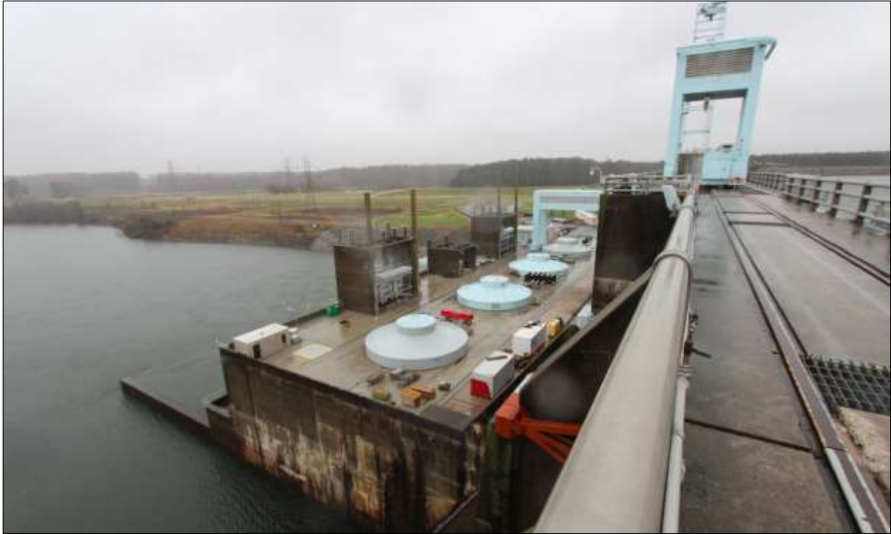
Figure 3.8. Cowans Ford Powerhouse from top of spillway, facing west.
